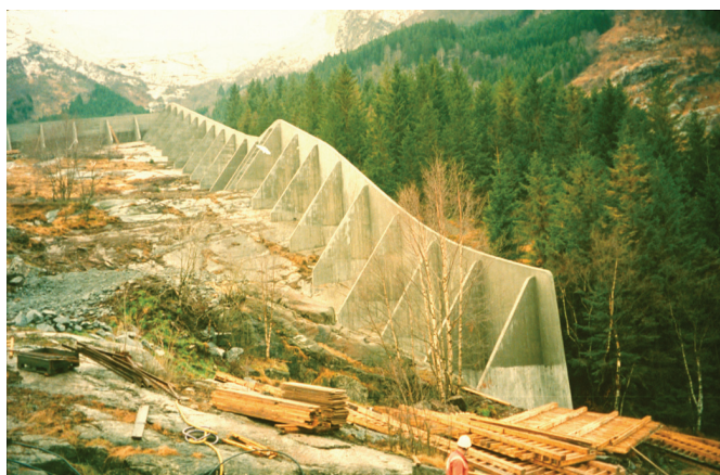
Figure 15.10: A concrete diverting dam at Odda, Norway (height 8 m, length 200 m) (photo: Karstein Lied).
