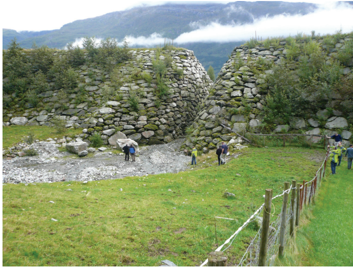
Figure 15.6: A river outlet trough a dam (photo: Karstein Lied).
