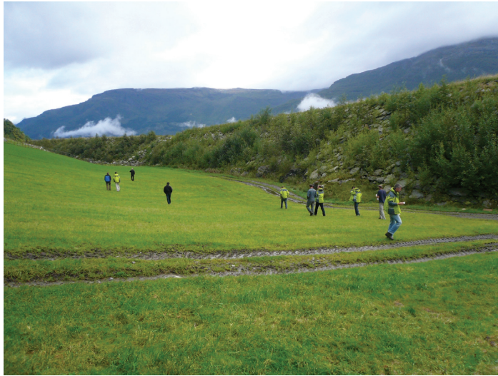
Figure 15.5: A catching dam for wet snow avalanches and debris flows. Dry wall with backfill of earth materials, height 12 m, inclination 1:1. Ullensvang, Norway. (Photo: Karstein Lied.)
